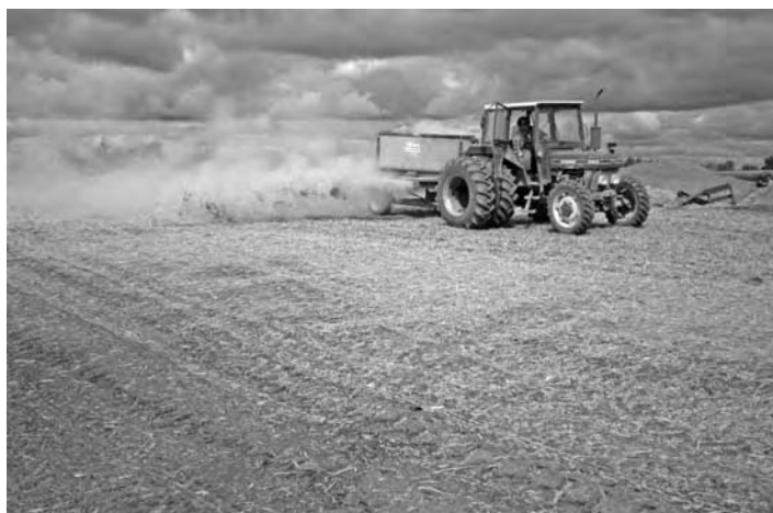
FIGURE 17.13 Agricultural-type seed bed preparation of tailings areas (photo by Inco, Ltd.).
