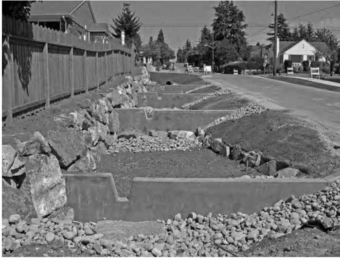
FIGURE 13.5 Check Dams on NW 107th Street in Broadview Green Grid increase retention time of storm-water on steep slopes (shown during construction). Photo by S. Hurley.
