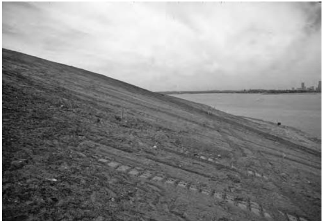
FIGURE 2.18 The soil profile in place on the upper north slope of the north drumlin, Spectacle Island.
