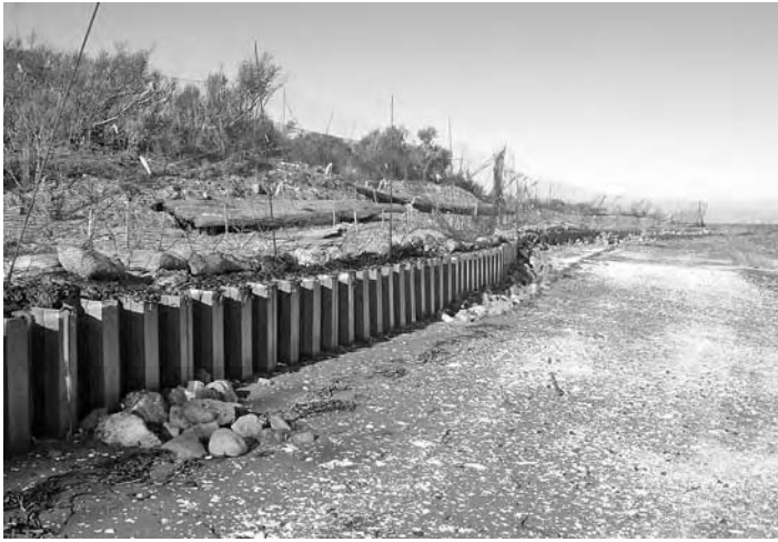
FIGURE 14.21 Erosion control structure to protect the Tuluwat Village Shellmound, Eureka, California. Note: Temporary deer fencing to protect native planting and additional cobble facing still to be installed. Photo by A. Davis (2006).
