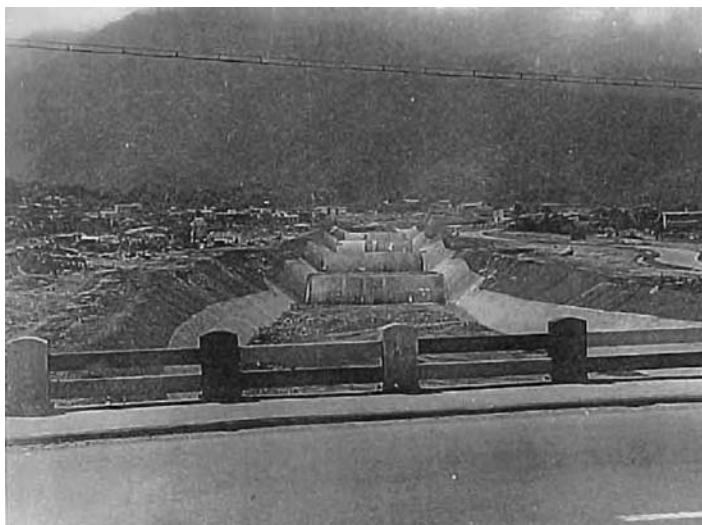
FIGURE 16.11 Cement lined channels have constrained mudflows, and instilled a false sense of security which has resulted in urban development adjacent to the channel environment. (Color version available at www.gsd.harvard.edu/restore .)
