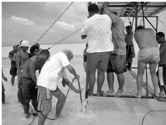
FIGURE 7.11 Jetting solar panel into the sand with a SCUBA tank on Helen Reef, Palau.
