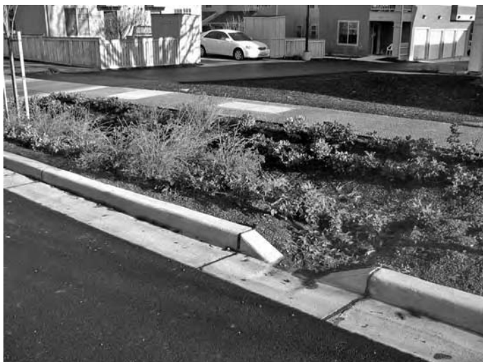
FIGURE 13.15 Curb cuts allow stormwater to flow from roadway into vegetated swales at High Point. Photo by Eric Higbee.
