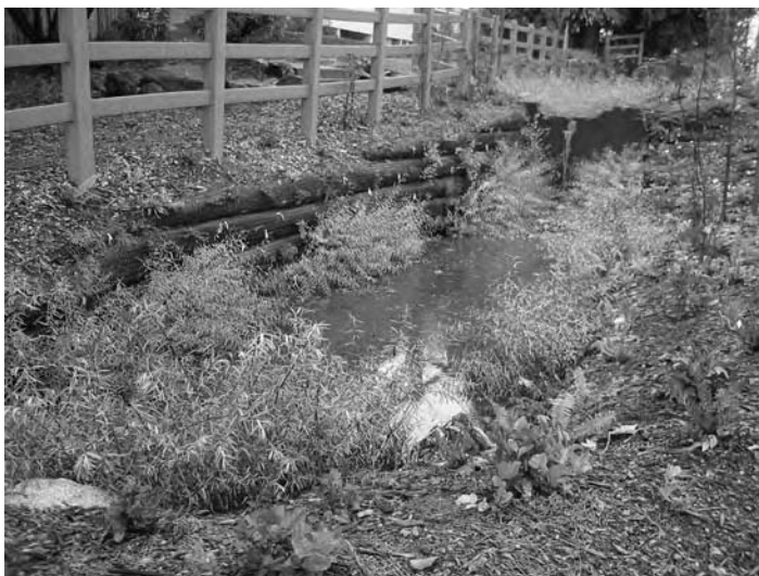
FIGURE 13.6 Willows were planted into “soil-wrap” walls that line the swale systems along NW 110th Street. Photo by S. Hurley.
