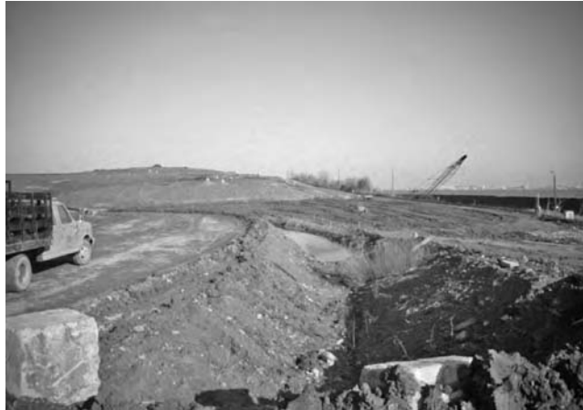
FIGURE 2.8 A view of a portion of Spectacle Island during placement of excavated fill and residual island subsoil.
