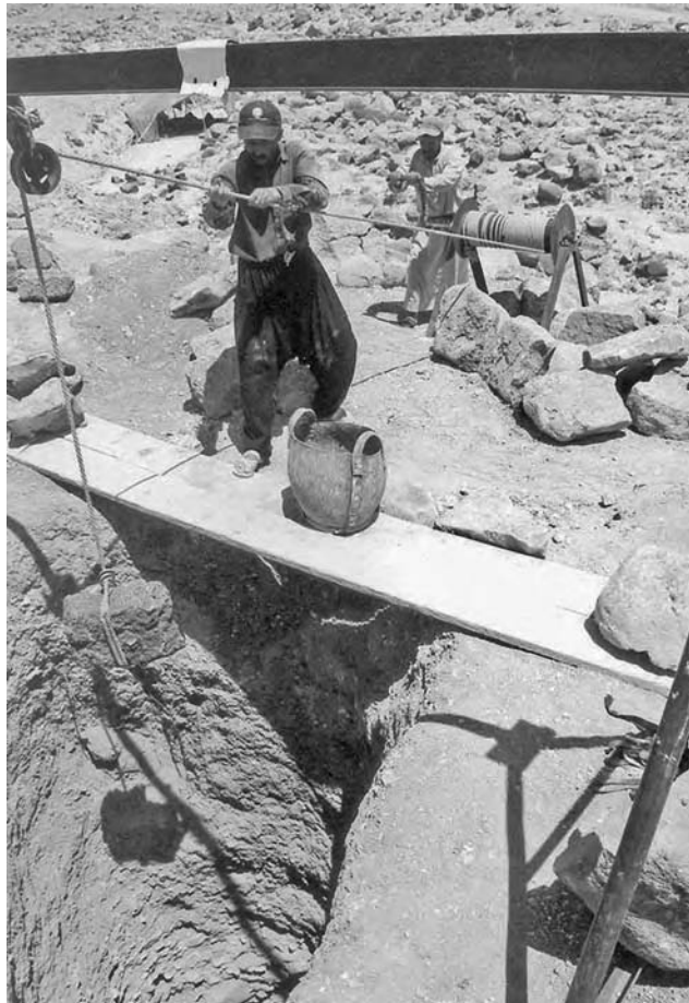
FIGURE 11.10 Renovating an airshaft of the qanat in Shallalah Saghirah.
