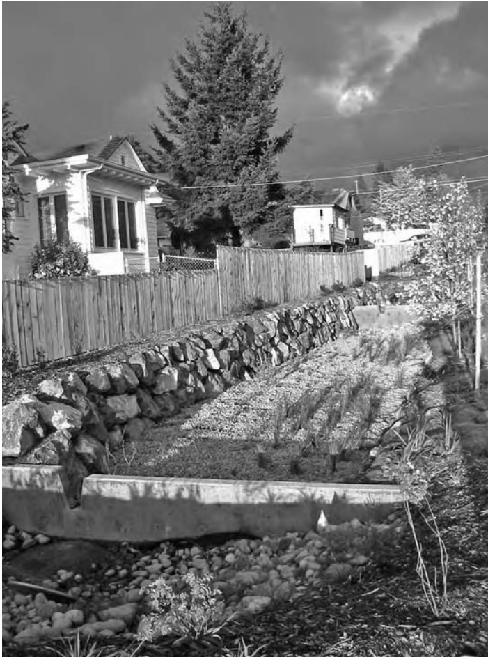
FIGURE 13.7 Rockery walls were used to reinforce the swale side-slopes along NW 107th Street in Broad-view Green Grid. Photo by S. Hurley.
