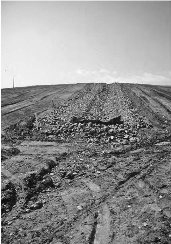
FIGURE 2.22 Rip-rap erosion control swale constructed by the contractor, Spectacle Island.
